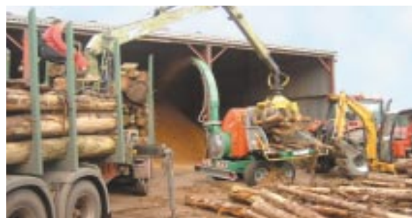
Chipping wood from local woodlands. Image: Marches Wood Energy Network
