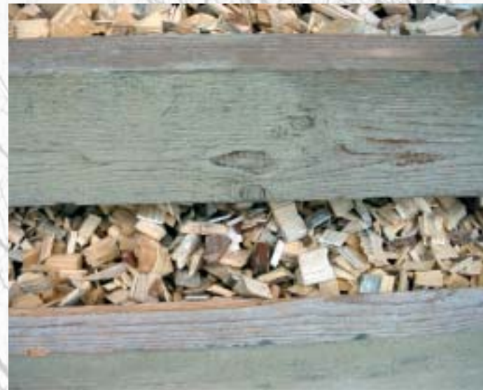
Quality chips matched to the boiler are vital.
